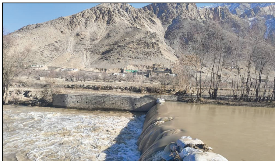
Figure 13: A low-height diversion dam on the Logar River, supplying water to the Joee Mastan canal. The dam's limited height restricts sufficient water diversion, underscoring the need for improvements to enhance water flow and distribution.
